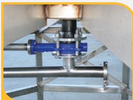
Flange fittings with butterfly valve
